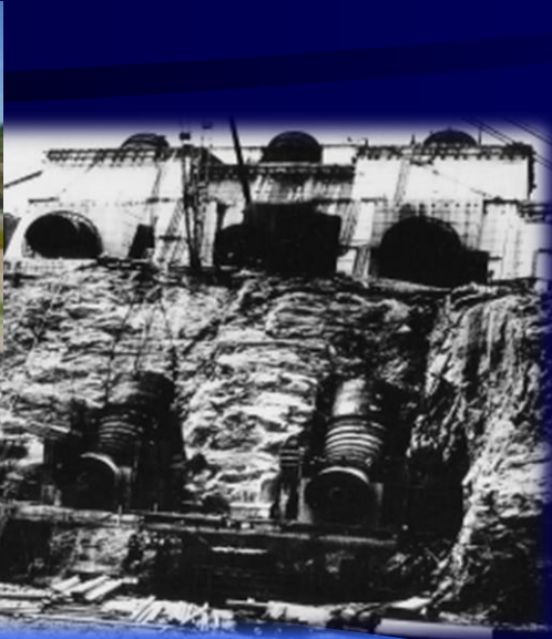
Penstocks at Raul Leoni en Guri Dam
