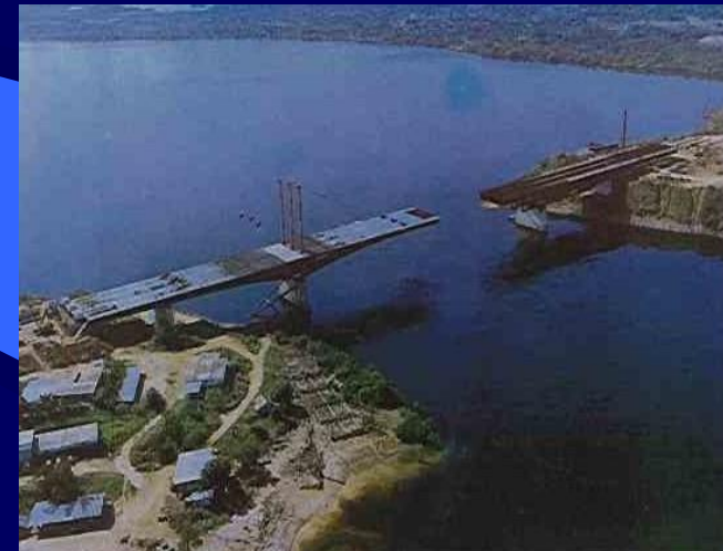
RAILROAD & HWY BRIDGE OVER CARONI RIVER
