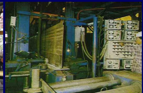
Automatic SAW Beam Welding
