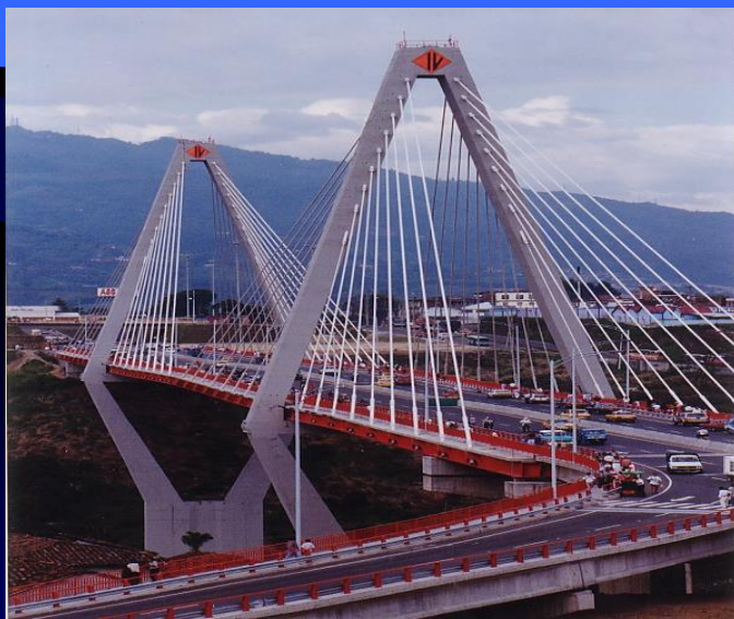
PEREIRA CABLE STAYED BRIDGE COLOMBIA
