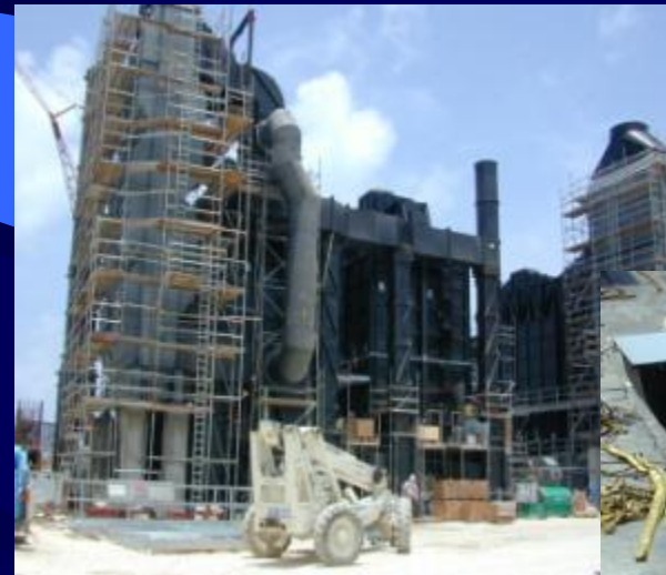
Ducts Plate Work
